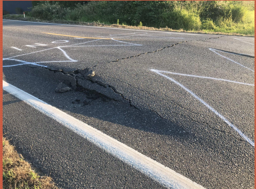
Trooper Kelsey Harding (@wspd7pio). (2021, June 28). State Route 544 milepost 7 near Everson, Wa is currently closed. The asphalt roadway is buckling and unsafe for travel. WSDOT is advised and detours are currently being set up. BL https://t.co/5Yb9UYzbDc [Tweet]. Twitter. https://twitter.com/wspd7pio/status/1409353681287592970
